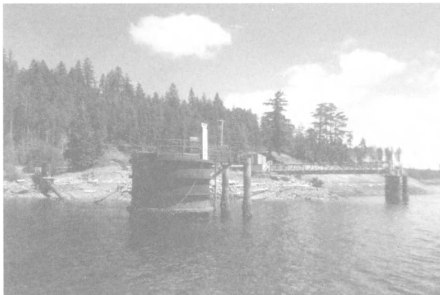
Fig. 9.5. The tailings outfall at Island Copper Mine. De-aeration/seawater-mix tank is shown in foreground . The tailings input line to the tank is visible on the shoreline to left at point of descent underwater. Not shown is the tank output line which descends to 50-m depth. The original outfall, with input by open flow, is shown right , and remained operational as a standby
